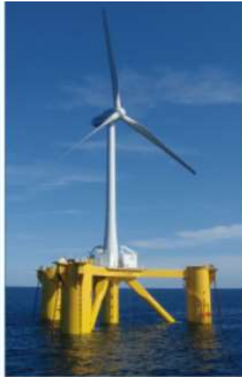
Compact semi-sub 2MW
