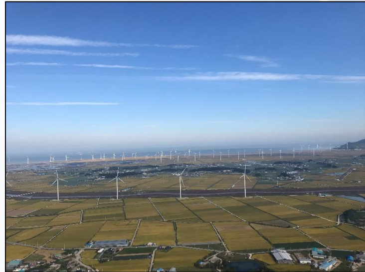
[Commercial 34.5MW] Unison 2.3MW x 15units (Jeonnam Yeonggwang) onshore&offshore complex
