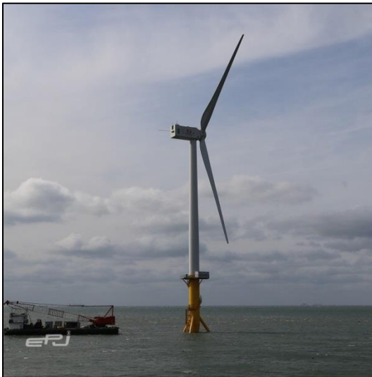
[Proto Type 3MW] DHI 3MW Suction bucket Type (Jeonbuk Gunsan)
