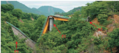
Fig. 3. (a) Sketch of collapsed Matsurube Bridge [22] and (b) in-situ photograph [23].
